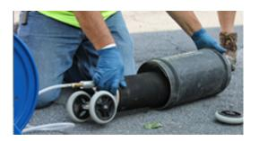
**RauschUSA offers Quick Lock Point repair systems** and supplies. Quick Lock is a strictly mechanical point repair system for the inside repair of pipes. No resin is involved. This revolutionary system consists of only (2) components: a 316L stainless steel sleeve structural body, covered by a seamless EPDM compression seal. Call us for systems information, we also sell the supplies if you are already set up.
